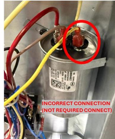
During Installation or motor replacement review the wiring diagram. Do not connect the outdoor fan motor yellow wire to the capacitor on these listed models.
