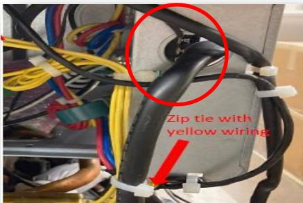
7. Plug in the wiring harness from the drain pan heater into plug X294 on the A2P board.
